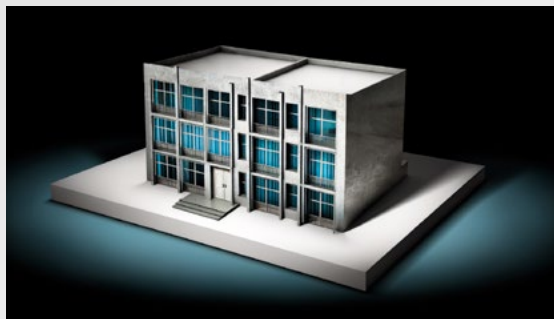
/ Protection FB6 Data center
